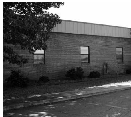
This recently-acquired facility in Sandy Springs will eventually house the College's Welding, HVAC, and Construction programs.
